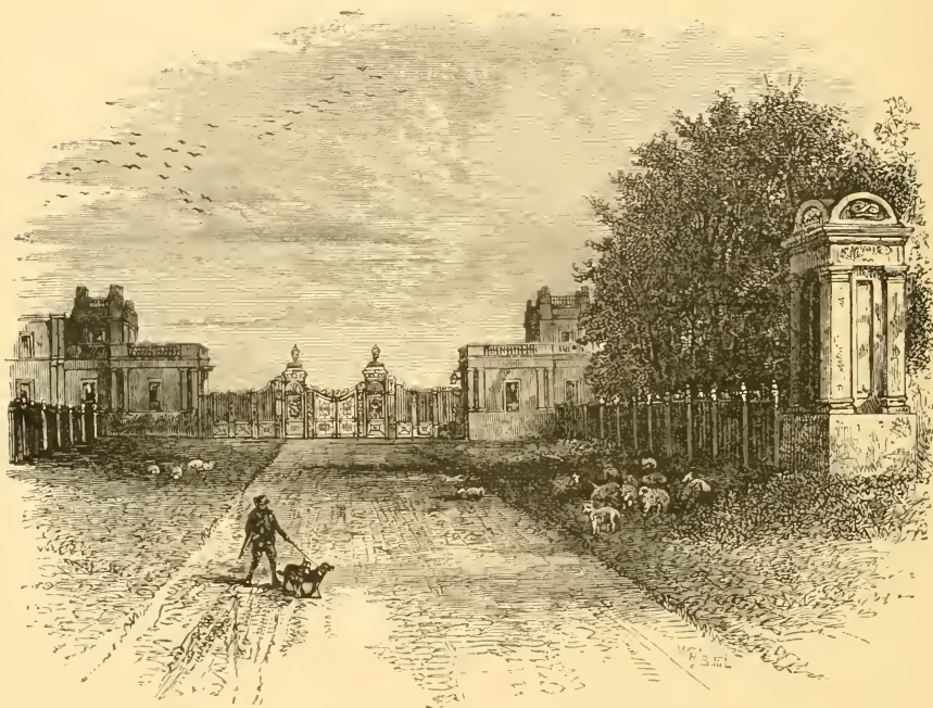
The Grand Entrance-Lodge at Baslow.
